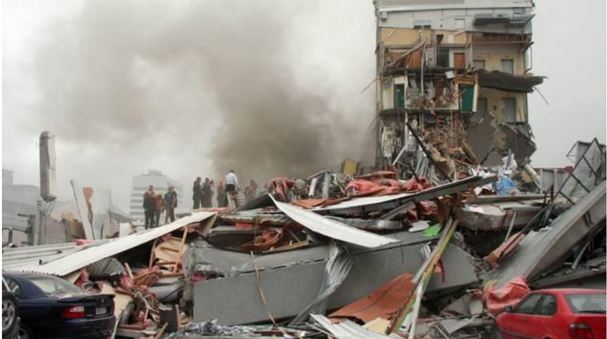
The CTV building. Photo / NZ Herald
